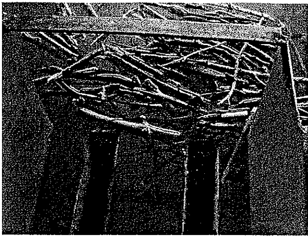
Figure 11. Operation of P.K. Weir with obstruction of the entry by floating debris.
